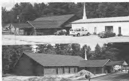
Front and back view of new facility
