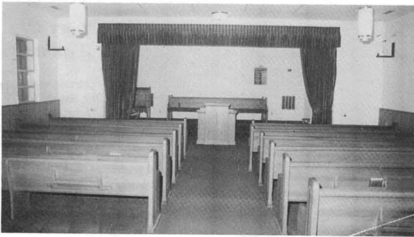
OLD SANCTUARY CONVERTED TO CLASS ROOMS AND CHILDREN'S CHURCH FACILITY
