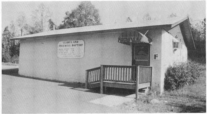
EXTERIOR OF CURRENT FACILITY
