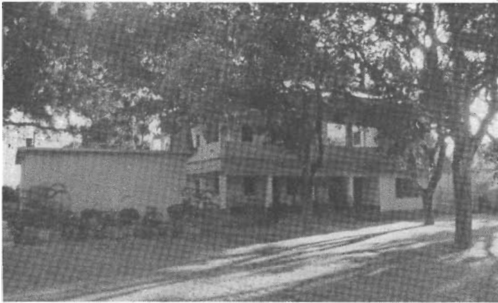
The Hostel Building That Now Houses 35 Children. It Is A Two Story Building Constructed of Concrete With Porches On Each Floor That Extend Completely Around The Living Area.
