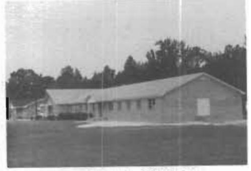
Grace Facilities With New Addition And Parsonage
