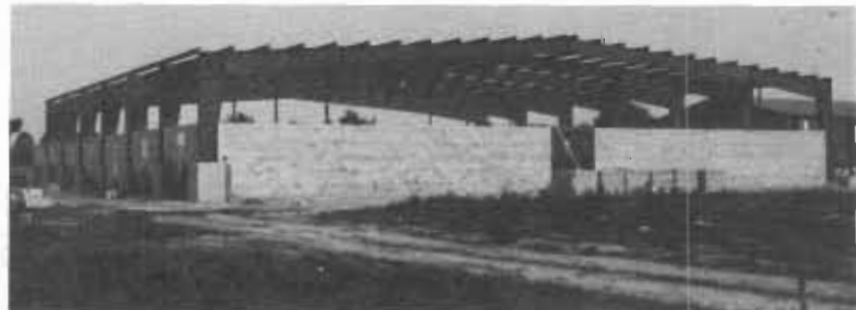
New Facilities For FFWB, Florence
