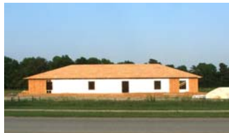
Framed and Roofed
