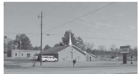
The new Fellowship/Educational Building is directly behind the Church
